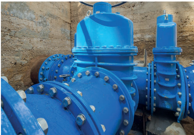
Large screws subjected to strong chemical aggressions, oils and stressed due to aggressive environment.
